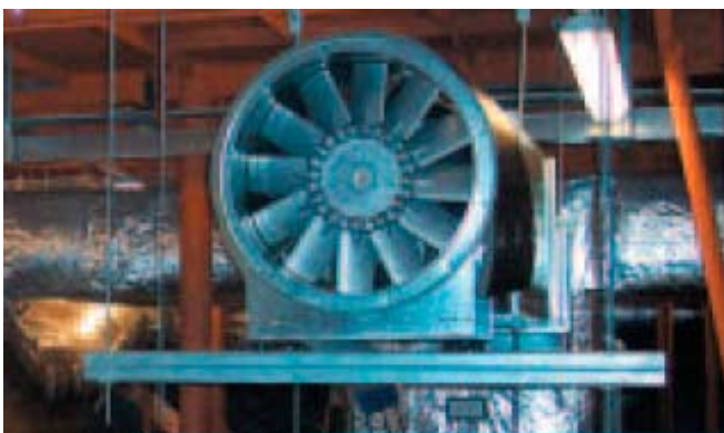
Dehumidification ducts being installed aboard the restored SS Great Britain.
