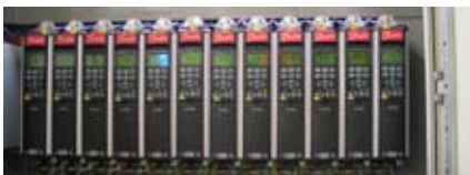
Real side by side mounted VLT® drives
